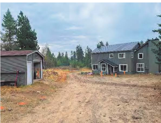
future carport site (bldg. approved)
