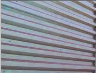
BRIDGER STEEL BOX RIB 7.2 STRUCTURAL SIDING COLOR DARK GRAY OR SIM.
